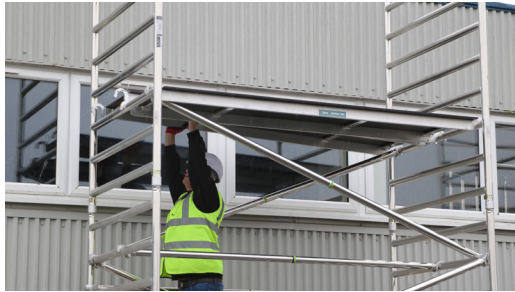
16. Fit your working platforms on the 6th rung ensuring the trap is opening outwards to the tower and inlin with the trap platform below. If needed, reposition your temporary board from below.
