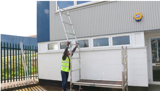
6. Add further frames ensuring the ladder is continuous.
