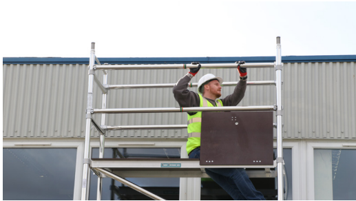
16. From a seated position, using the 3T method, fit 4 horizontal braces above the appropriate rungs to the frame vertices, hooks facing out.
