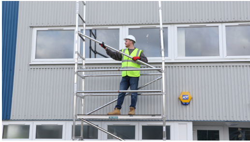
14. Continue erecting the tower fitting the frames and diagonal braces as illustrated using all components. Platforms inserted every 2m complete with handrails. Braces run in a continuous pattern on opposite sides except where interrupted by a platform. Then braces can be stepped up/down 1 rung.
