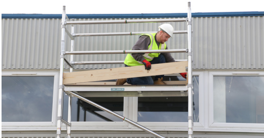
17. Fit toe-boards in correct position
