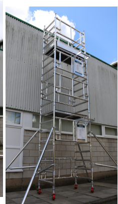
4.1m Tower Set up
