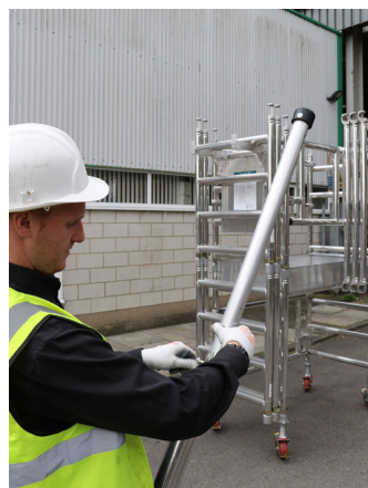
18. Before fitting stabilizers, release the pin to enable extension.
